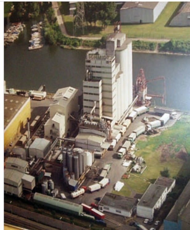
Cargill's heat exchanger plant demonstrates good practice in energy use and pollution control
