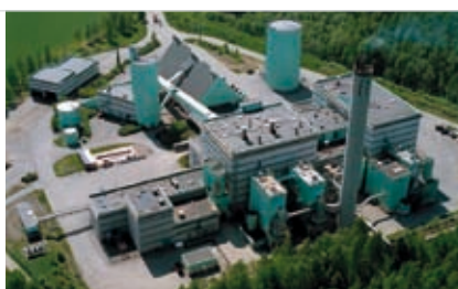
The Biomal plants' simple and effective approach holds strong demonstration value for other Member States
