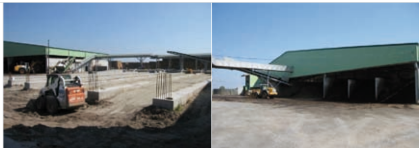
24 compost tunnels were constructed by the end of 2007
