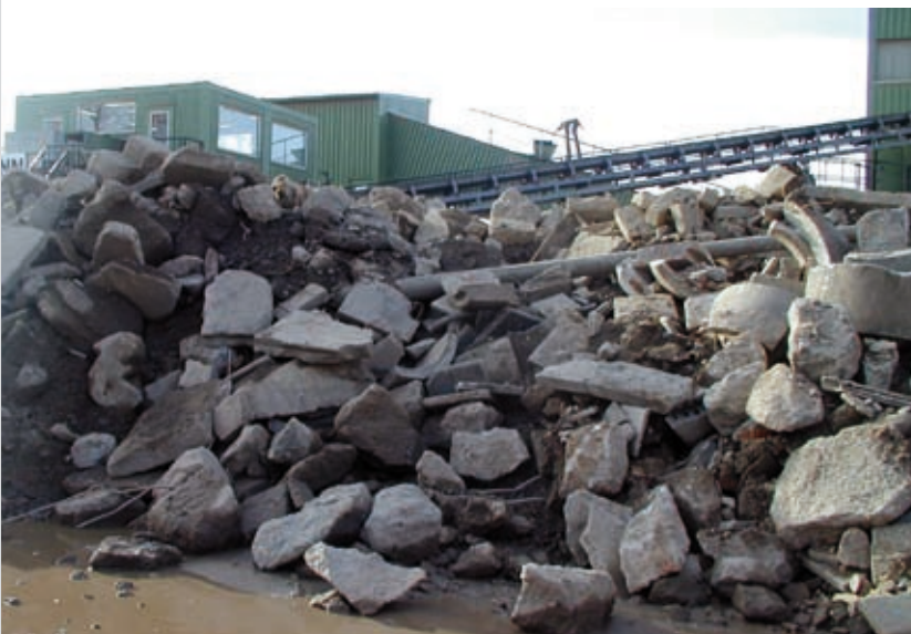
Concrete rubble before dry treatment
