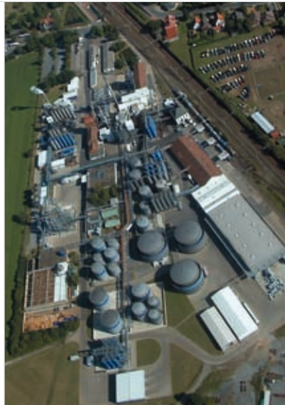
Aerial view of the Mineralöl-Raffinerie Dollbergen site
