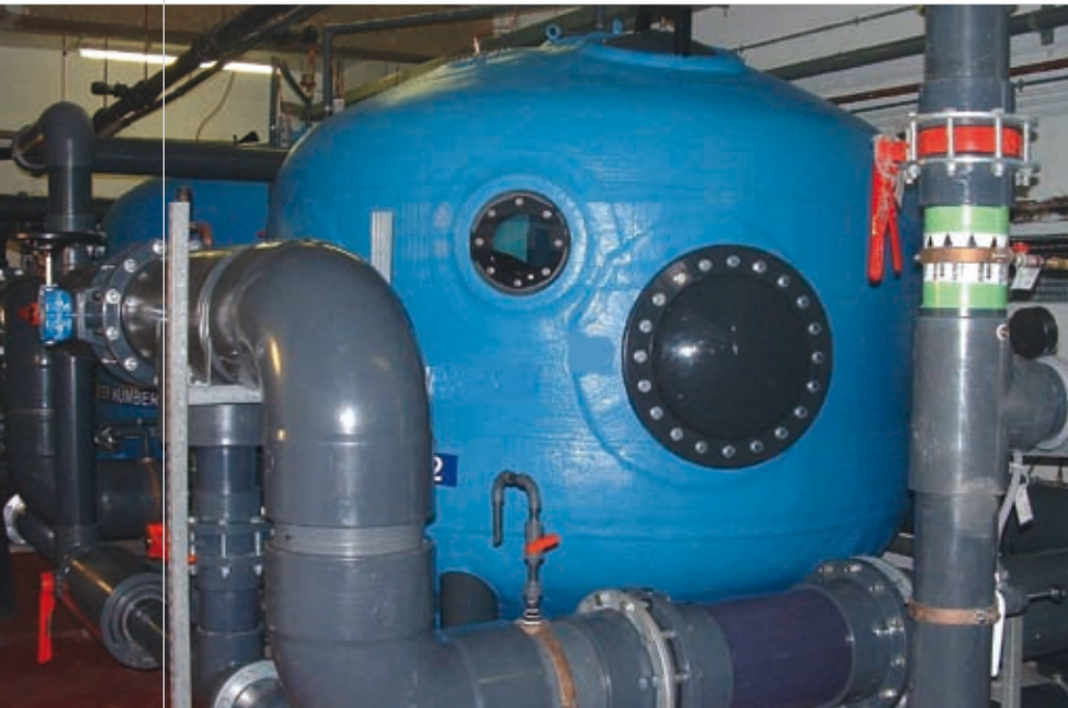
Recycled glass is the basis of the water filtration medium used here, in this Scottish swimming pool
