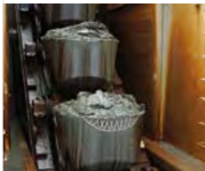
Removal of TBT contaminated sediments
