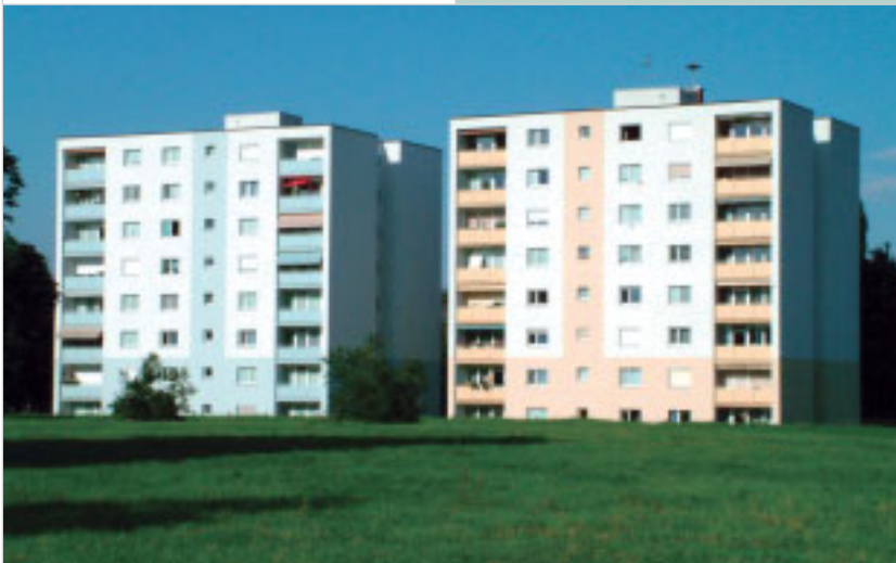
Kappelerstraße in Graz, after renovation work.
