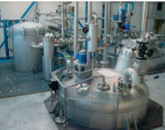
The installation of the filtration unit (shown here) made it possible to re-use the spent rinsing MMA twice before sending it to distillation. This resulted in a 50% reduction of the waste stream.
