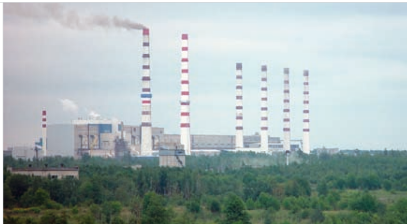
The Balti power plant is one of the largest oil shale-fired power plants in the world.
