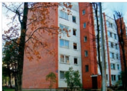
The 139 multi-storey apartment buildings were energy-rated.
