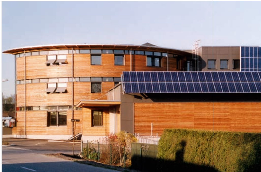
The Christophorus House consumes 275,000 kWh annually less than other buildings of its size.
