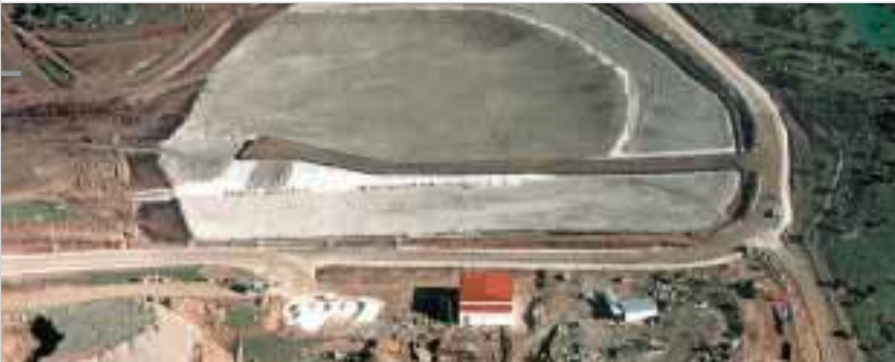
Building a waste treatment plant in Larissa.
