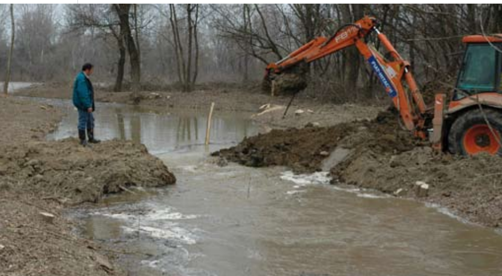
The floodplain's water retention capacity was expanded through the excavation of borrow pits and the opening of flood channels
