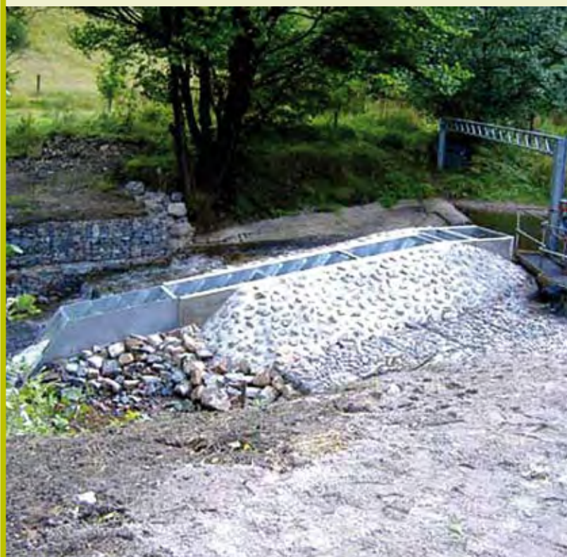
Removing river obstacles by building a fish passage
