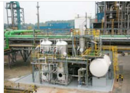
The brine recovery finishing unit was made up of salt removal columns and a carbonate destruction system
