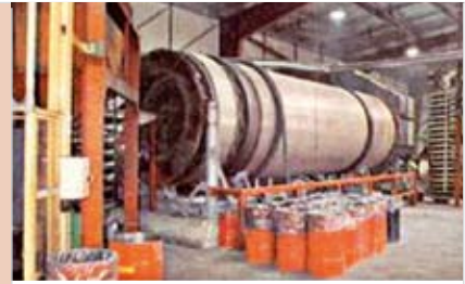
The regeneration of used catalysts is carried out in a modified furnace that restores the catalyst's original properties
