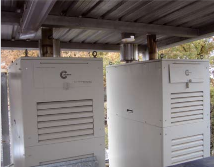
Two 30 kW microturbines were installed on the Orís landfill and operated successfully with gases with methane levels of 35% or lower
