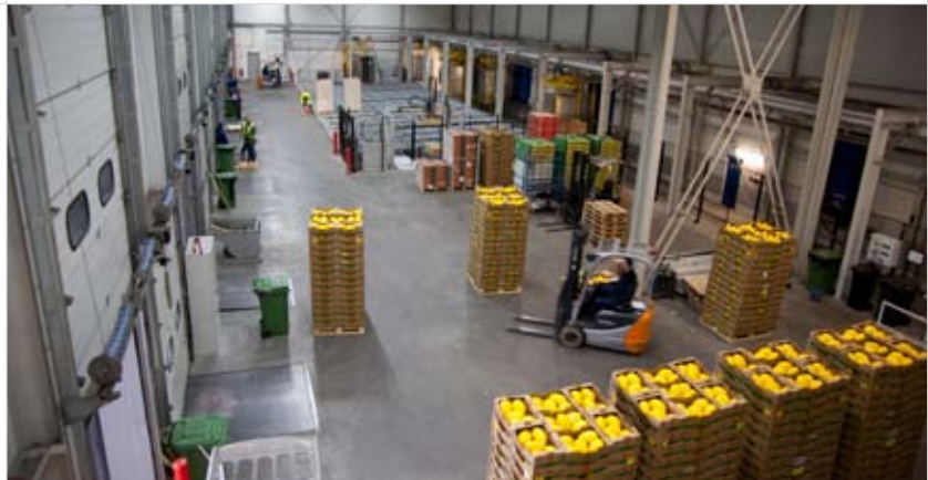
The HEIGHT project demonstrated that a high rise cold store using ammonia and CO 2 technology offers energy savings of around 75% compared with conventional cold stores
