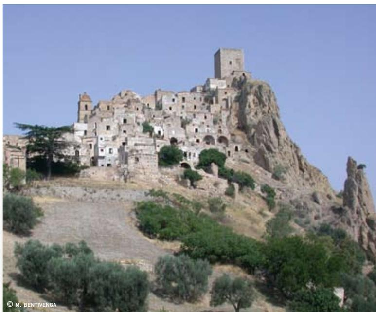
Fig. 6: Craco, built on a limestone base (calcarenite) sitting on extremely uneven clay formations, which have caused the instability of the foundations of the settlement.
