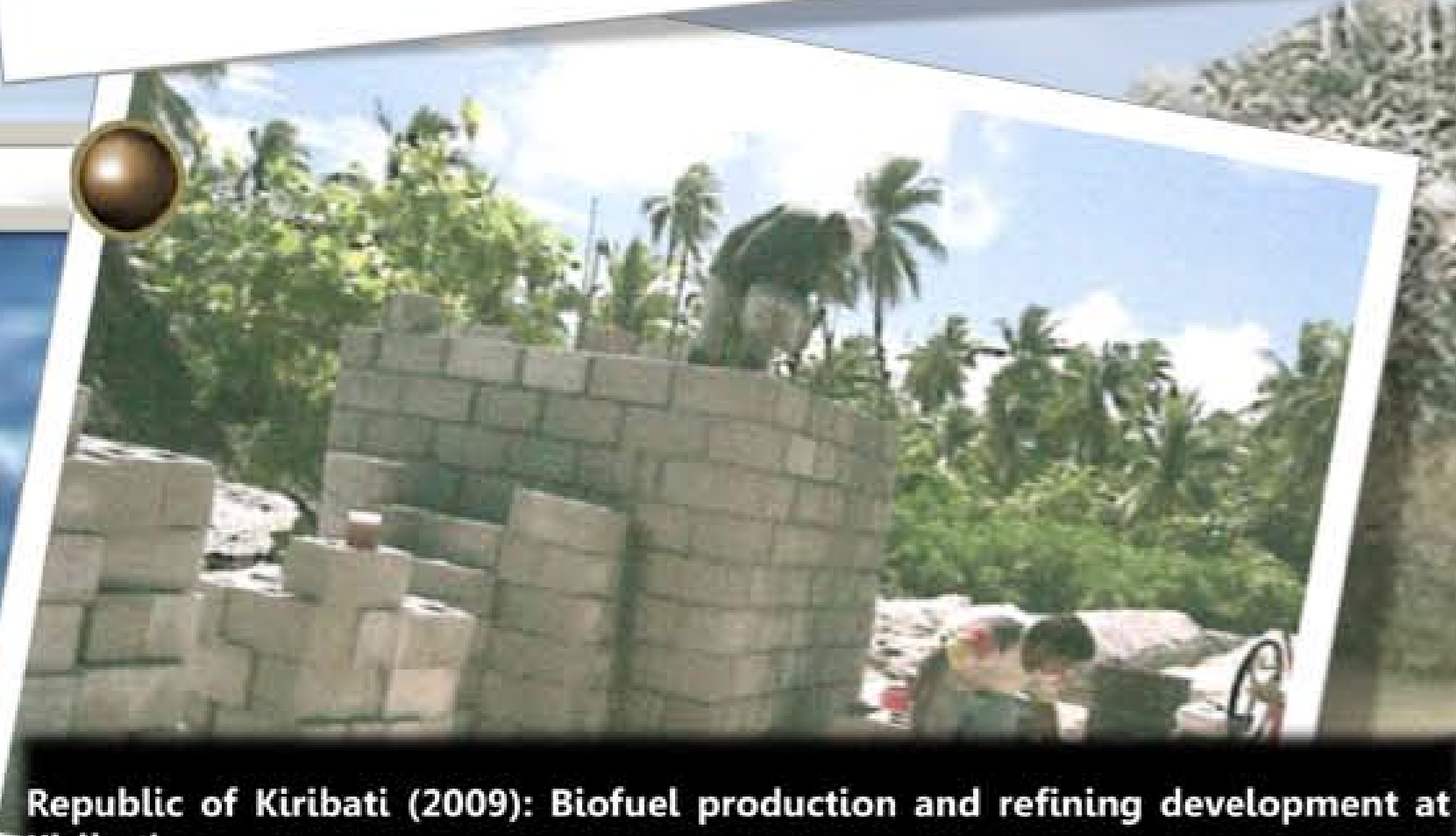
Republic of Kiribati (2009): Biofuel production and refining development at Kiribati A biofuel plant was installed to produce fuel from Coconut oil supplying transport and electricity generation sectors on the island.
