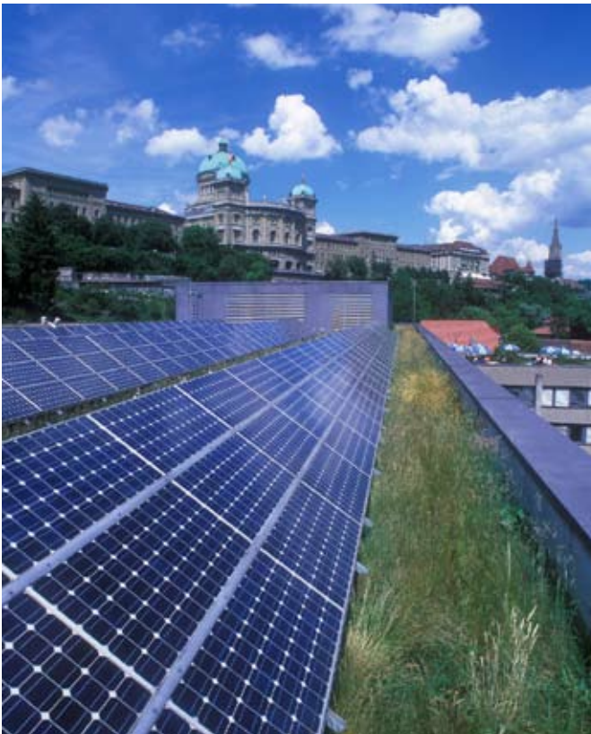
© Martin Bond / Still Pictures Arrays of photovoltaic cells on the roof of a government of ce building. In background, Swiss federal parliament buildings. Berne, Switzerland.
