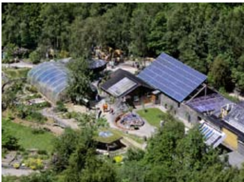
© Martin Bond / Still Pictures The Centre for Alternative Technology, showing polytunnel, geodesic dome and on the right, a photovoltaic roof for generating electricity. Wales, near Machynlleth, UK.
