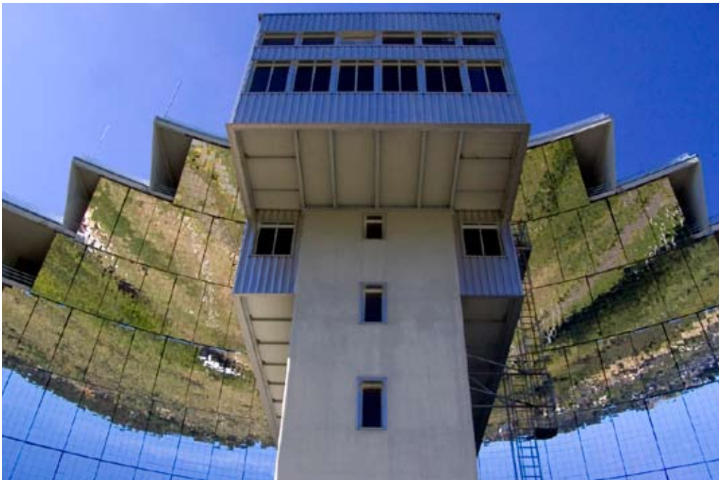
© T. Mohr / Still Pictures Solar thermal collector. Font-Romeu, France.
