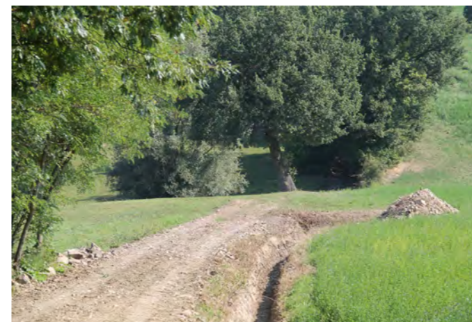
RATIONALIZATION 3: CLEANING AND REMODELING OF DRAINAGE DITCHES
