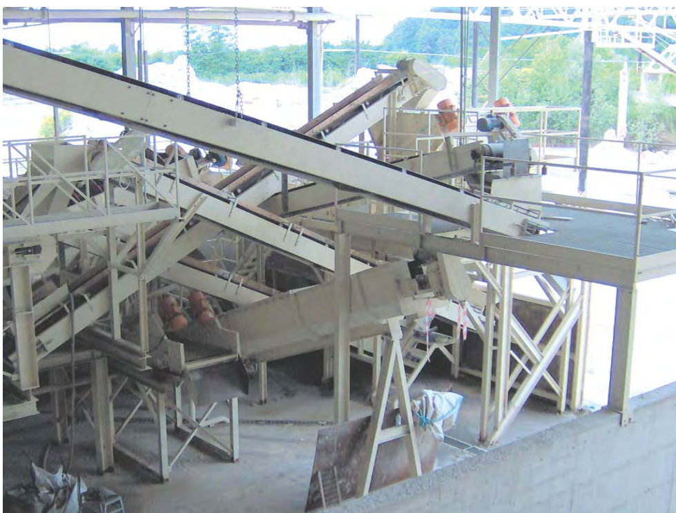
Figure 1 - View of material treatment plant
